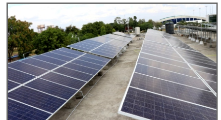
120 KW Airport Authority of India, Aurangabad, INDIA
