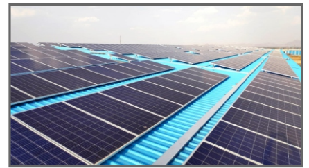
400 KW HTL Metals Ltd. Hindupur, Andhra Pradesh, AP, India.
