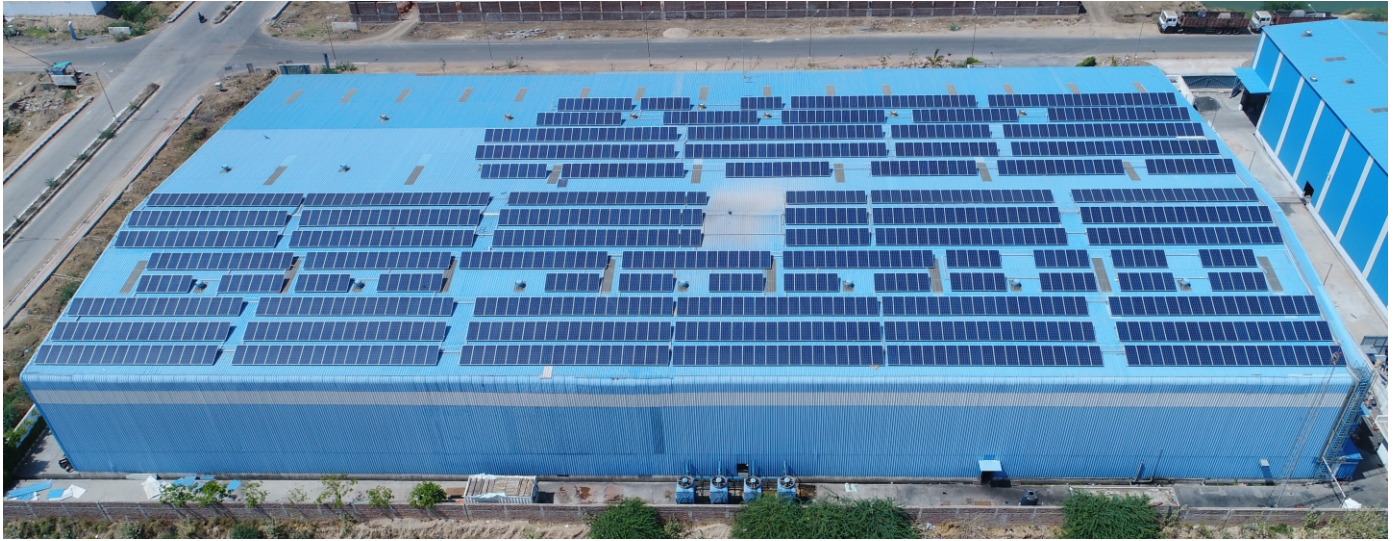
450 KW Hi-Tech Pipes - Sanand
