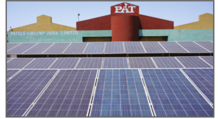
130 KW Patel Airtemp, Santej GIDC, Ahmedabad, Gujarat
