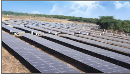
10 MW Jay Chemical Industries Ltd., Khambhat, ANAND, Gujarat
