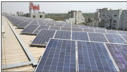
200 KW AmulFed Dairy, Bhat, Gandhinagar, Gujarat
