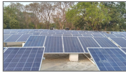
200 KW IOCL, Gujarat Refinery Twp, Karachiya, Vadodara, Gujarat.
